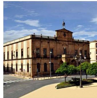
SOLAR PV SKYLIGHT - LINARES CITY HALL
