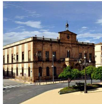
SOLAR PV SKYLIGHT - LINARES CITY HALL
