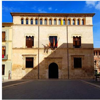
SOLAR PV SKYLIGHT - ALZIRA TOWN HALL
