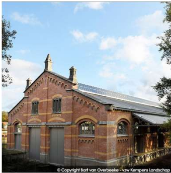
SOLAR PV SKYLIGHT - CUSTOMS WAREHOUSE
