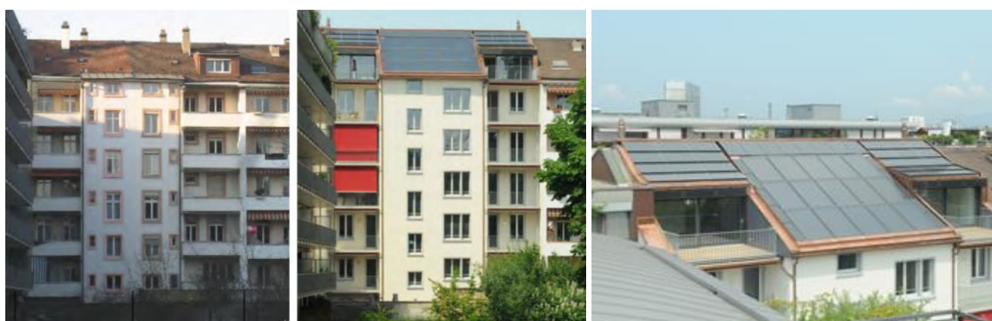
Figure 3: MFH-Multi-Family House, SanierunG Feldbergstrasse 4+6 BS (CH). Refurbishment of two houses in the protected area of Basel-Stadt. The solar roof on the south side provides more energy than is necessary for heating and hot water (Source: Swiss solar prize 2009, Viridén+Partner AG Zurich)
