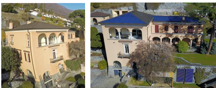
Figure 2: The 1939 built residence Villa Carlotta in Orselina / TI (CH), was recently renovated. The old oil heating has been replaced with a 38 kW heat pump solar-powered (BIPV in roof) with six geothermal probes ranging from 140 to 165 m in depth. The entire 350 m 2 roof area was equipped with a 51 kW PV system which covers the total energy requirement 87% (Source: Swiss solar prize 2018)
