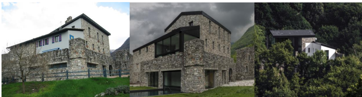
Figure 5: The refurbishment and addition of new building in the Doragno Castle, Rovio / TI (CH). It uses a BIPV on the roof (16'000 kWh/y), testing an innovative and sustainable solutions for multifunctional building envelope to achieve NZE standard, using ST and PV modules (Source: deltaZERO SA Architects, pictures Luciano Carugo)
