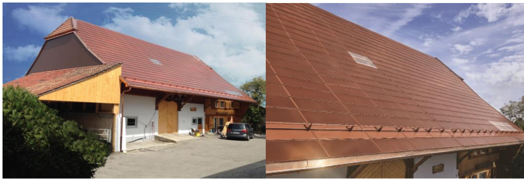
Figure 4: The Ecuwillens / FR (CH) rural house pilot project, dating back to 1859, uses clay-colored modules developed by the CSEM and Issol for sites protected by cultural heritage (Source: Swiss solar prize 2018)
