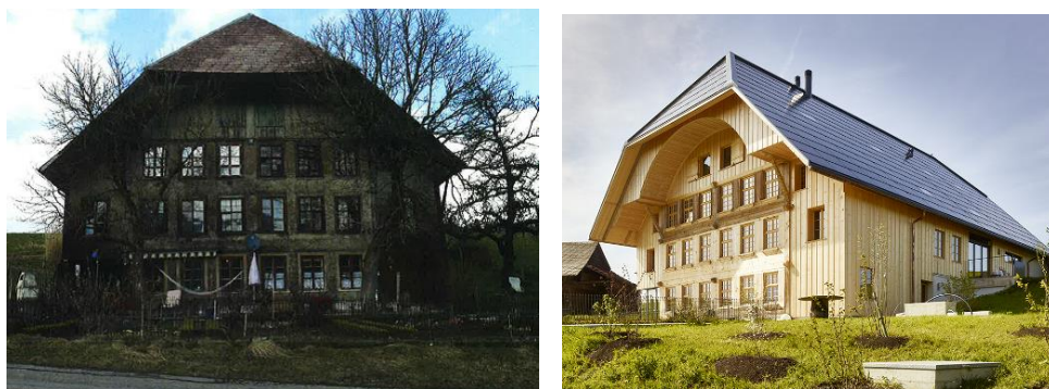
Figure 1: Example on solar BIPV integration in a Glaserhaus, built in 1765 in Affoltern in the Emmental / BE (CH). Left picture shows the front view of the house from 1765, in the last decades mostly uninhabited before the renovation. Right picture the illustrates the Plus Energy renovated building using BIPV solar technology in the roof, where tradition, modernity, sustainability and aesthetics complement each other and significantly improve the urban landscape (Source: Swiss solar prize 2016 and SUPSI-BFE database)
