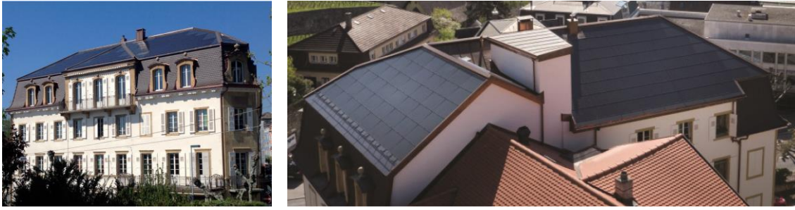
Figure 6: Hotel des Associations, Neuchâtel / NE (CH). The building is located in a ISOS protected area. Based on special and opaque modules, it integrates perfectly with the entire roof surface and preserves the historic character of the building (Sources: Swiss solar prize 2015).
